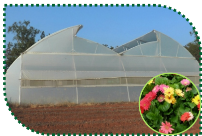
Naturally Ventilated Poly House
